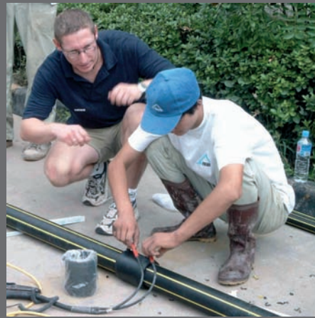
Demonstration of an electrofusion process. No questions remain unanswered when there is training on the construction site.
