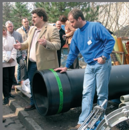
Seminars: The FRIATEC seminar leaders instruct the safe use of FRIALEN – even on site.
