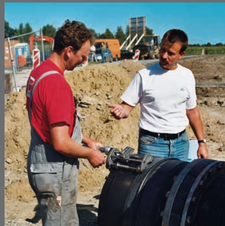
Advice on site: a FRIATEC specialist explains how to handle a FRIATOOLS scraper tool.
